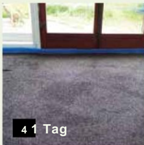
4 1 Tag Installation ThermoDyn substructure
