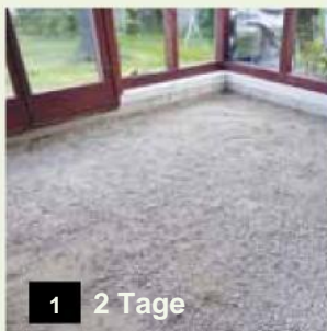
1 2 Tage Surface preparation
