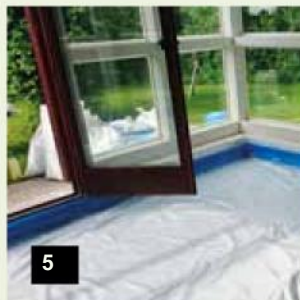
5 Installation vapour barrier
