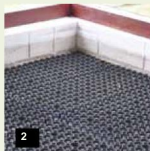
2 Installing the reinforcement grids
